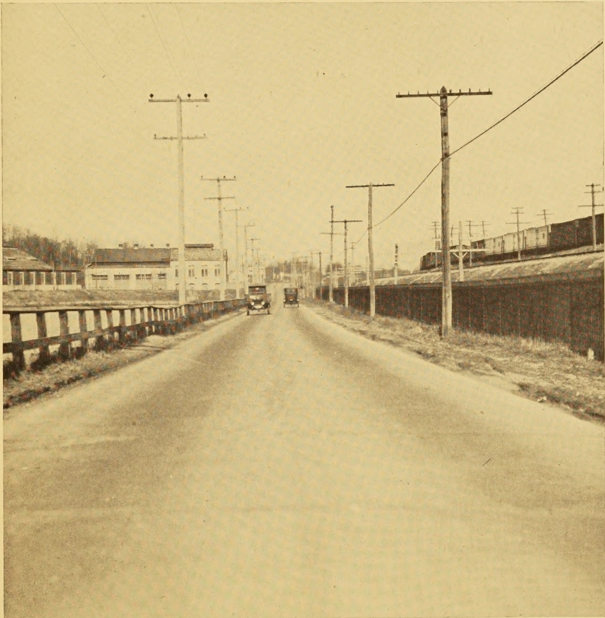
OIL STAINS ON A CONCRETE ROAD WHICH INDICATE THE LINES OF MAXIMUM TRAFFIC
